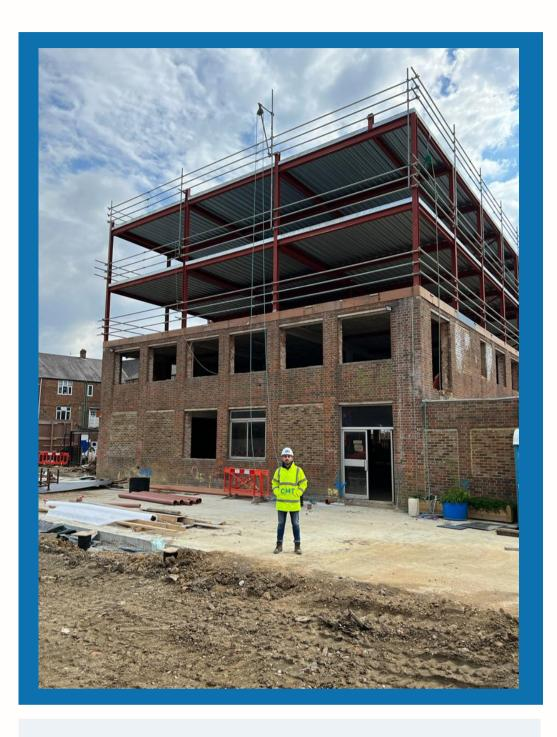
The project involves the change of use of existing building and third floor extension to provide a 66 bed hotel with complete internal and external refurbishment and reconfiguration. The building fabric will be updated and a new façade will be introduced to enhance the street scene and promote local distinctiveness.
